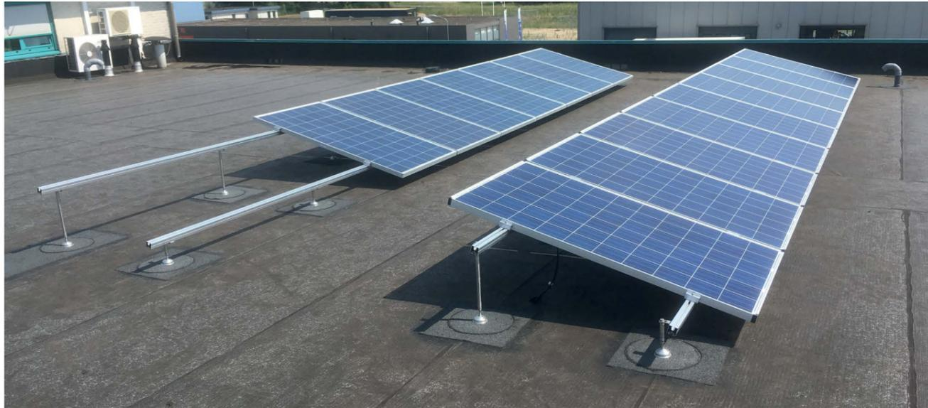
**Mounting anchors for ballast-free mounting systems.**
